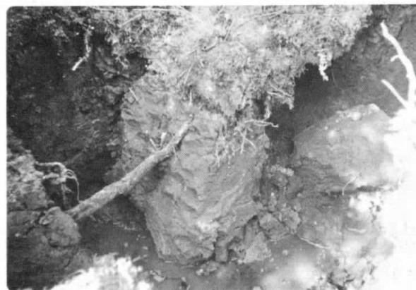
2. Soil mound, shored-up to prevent it from slumping into excavation.
